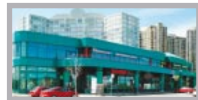
The New Ventures head office in Mississauga
